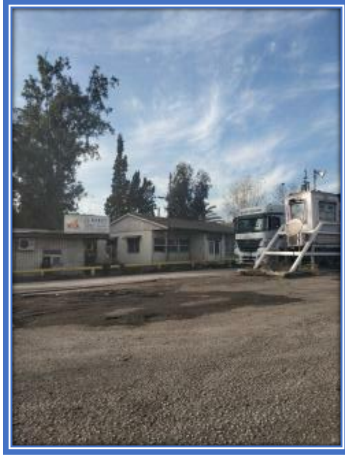
Figure 7-2 Structures in Toros Tarım I.C. Parking Area
